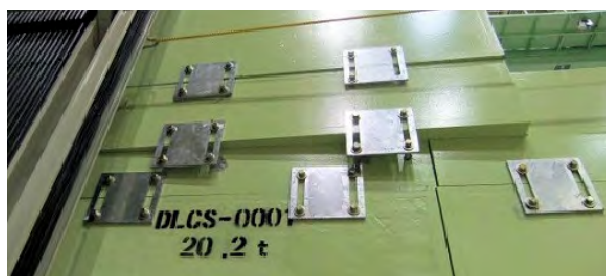
Fig.2: Concrete shield blocks above the secondary muon channel moved and broke the anchoring bolts.
