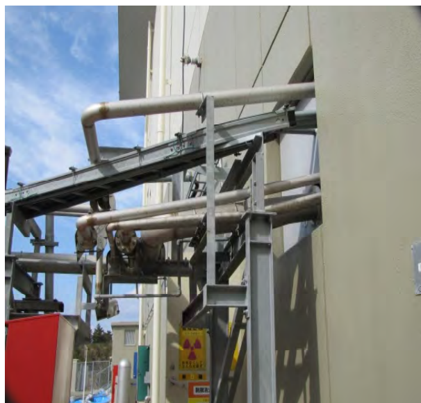
Fig.1: Outside the MLF experimental hall, the pipes to and from the compressor facility were bent and partly damaged the wall.
