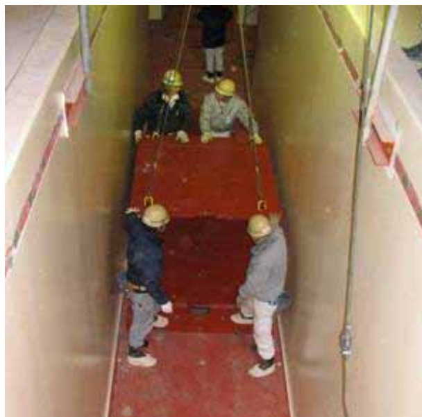
The alignment plates (red) placed on the floor of the M2 muon beamline at J-PARC.
