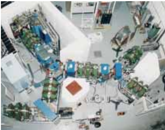
The RIKEN-RAL muon facility during construction.
