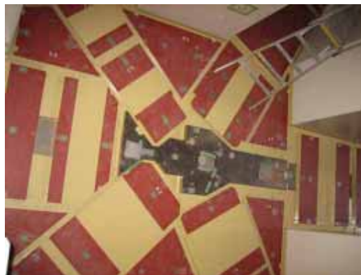
The alignment plates (red) placed on the floor of the M2 muon beamline at J-PARC.
