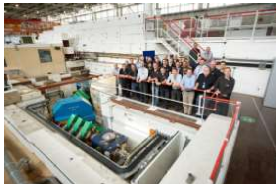
Fig ISIS2: The installation team for the beamline upgrade, with the new beamline in the foreground.
